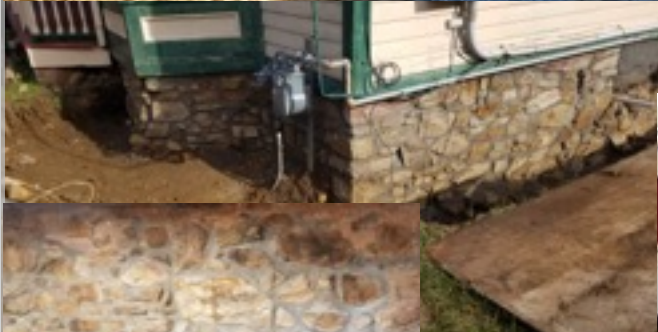
Repointed basement wall with ghost of old doorway
