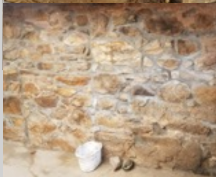
Repointed basement wall with ghost of old doorway
