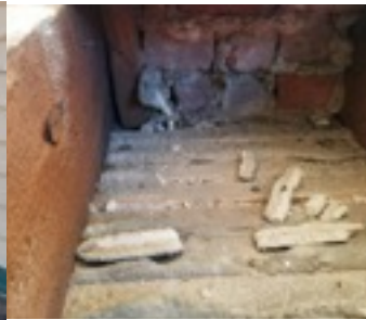
Above: unusual brick infill at the meeting of the second floor joists and outside wall
