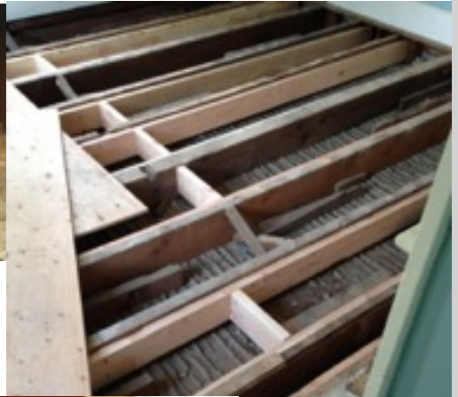
Above: unusual brick infill at the meeting of the second floor joists and outside wall
