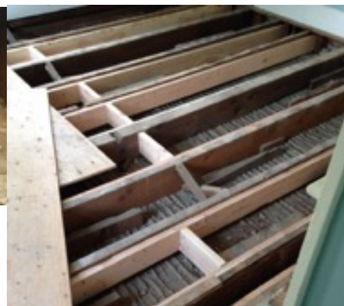
Above: unusual brick infill at the meeting of the second floor joists and outside wall
