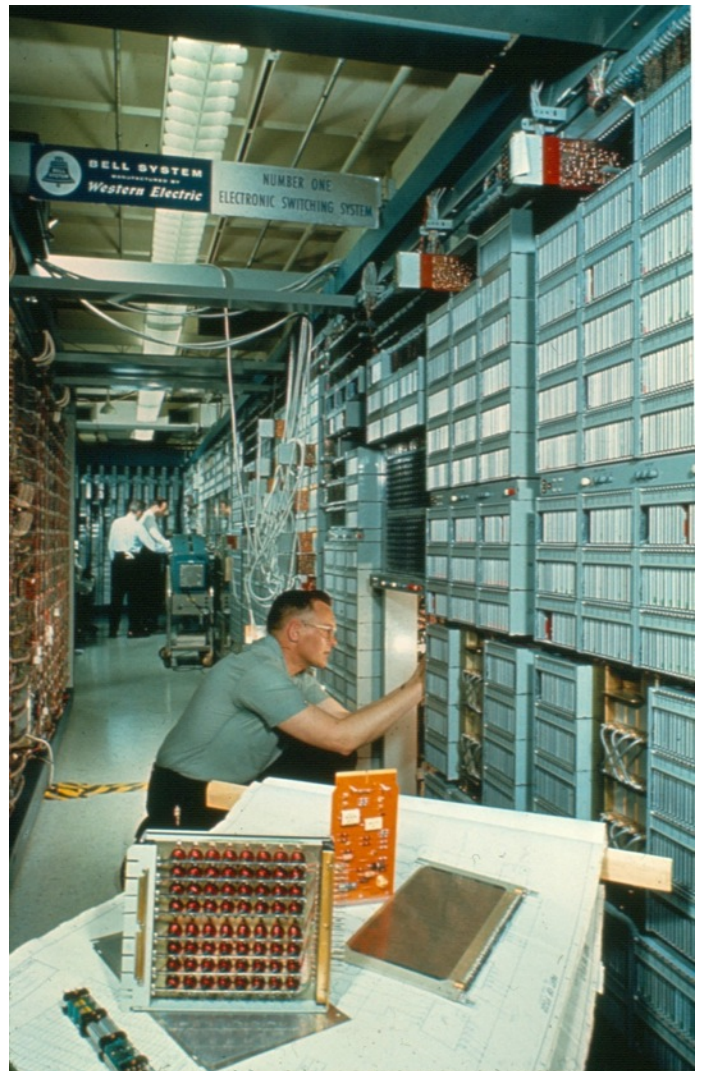
New Jersey Bell Switchman Fritz Blume checks circuit at ESS office in Succasunna, N. J. In foreground are some of the basic units of electronic switching left to right: dual sensor, permanent memory card, ferreed switch array, logic circuit pack (orange) and twistor memory sub-assembly.
